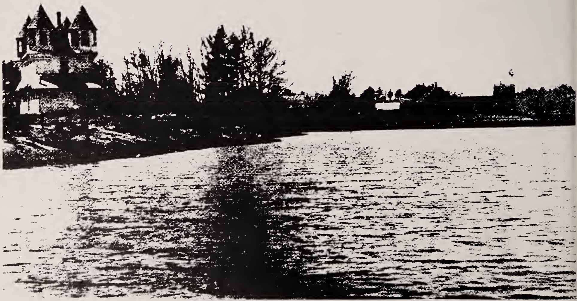
Hiller Laboratory and flooded Cranberry Meadow now the Masonic Hall and Rotary Park pond.
